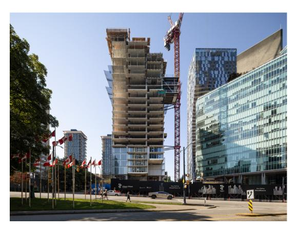
This entailed the on-site assembly of the structural steel components, followed by their lift into final position. Developed by Bosa Properties and Kingswood Properties, the 42-storey residential tower introduces a sculptural form to Vancouver's skyline, defined by bold cantilevers that project outward from the tower creating panoramic views of the city.
